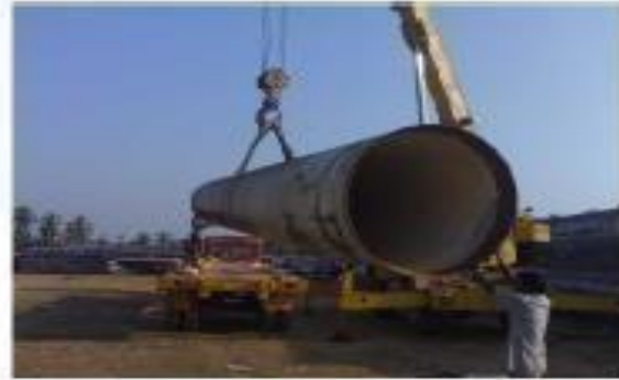
MS PIPE LINE UNLOADING - VEIAG STEEL PLANT
