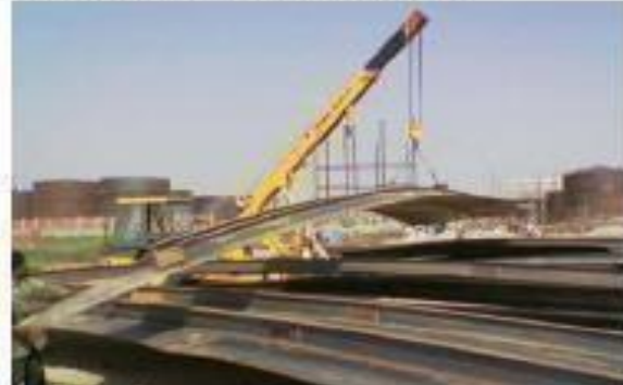
MS PLAT SHEDDING FOR TANK FABRICATION
