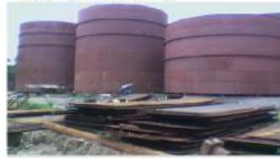
MS PLAT SHEDDING FOR TANK FABRICATION
