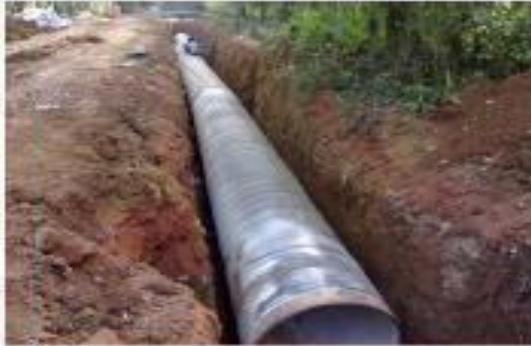
MS PIPE LINE WORKS FOR TPL - VEIAG STEEL PLANT
