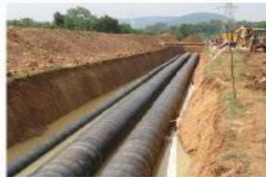
MS PIPE LINE INSPECTION FOR TPL DWARAKA SITE - VEIAG STEEL PLANT
